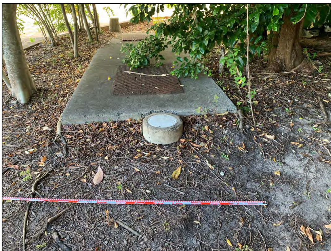
Plate 10: View north of exposed ground along western boundary showing services and introduced trees.
