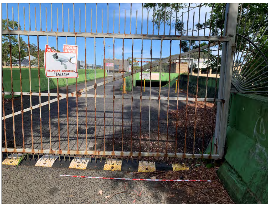
Plate 8: View west from Albany Street North across the north east portion of the study area showing derelict shopping complex with ramp to car parking below.
